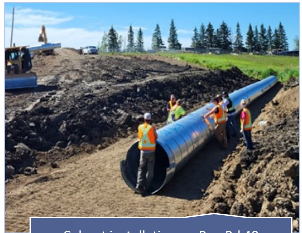
Culvert installation on Rge Rd 40
